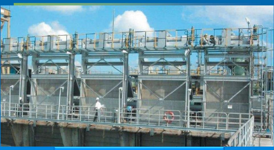
Mainly Used for SWRO Plants with Deep Intakes Distance Between Bars – 3 to 10 mm
