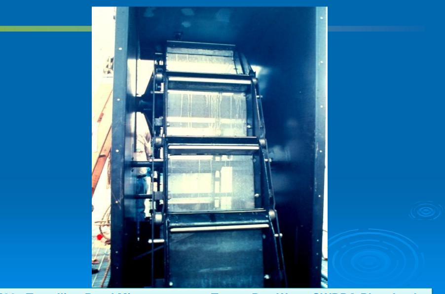
500 µTravelling Band Micro-screens – Tampa Bay Water SWRPO Plant Intake
