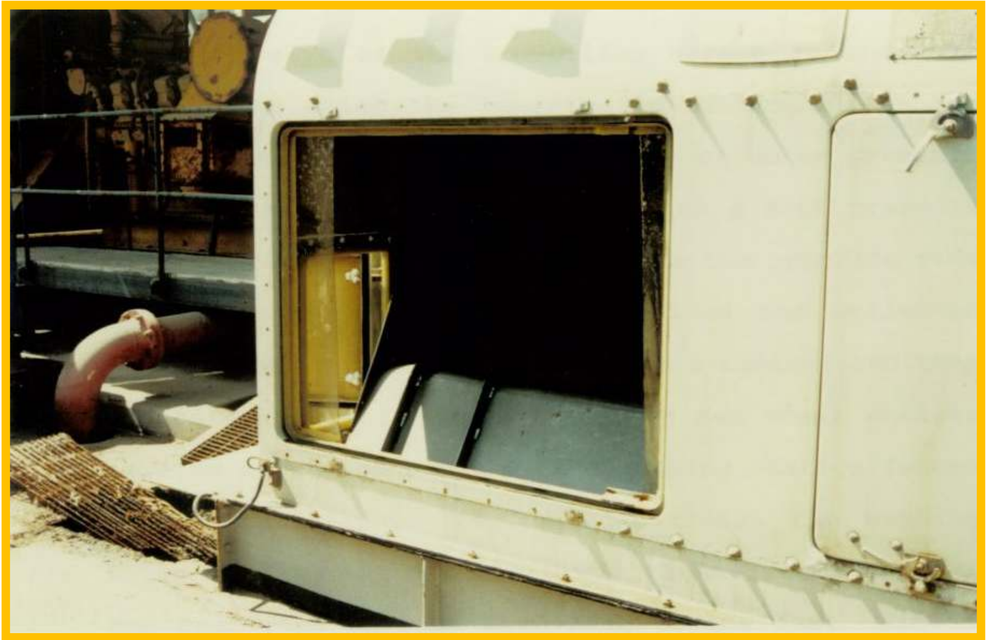
Housing of traveling screen mesh of <1\text{cm}^2
