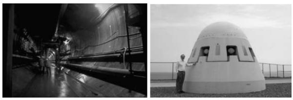
Figure 22: Boston outfall during installation in 1998. *Left*: View into tunnel section (16 km with 8 m diameter). *Right*: One out of 55 riser caps with eight outlets each in rosette-like configuration (Roberts and Snyder, 1993)
