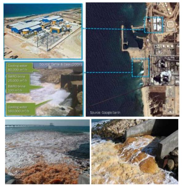
Figure 15: Ashkelon (Israel), RO plant with negatively buoyant brine discharge during backwash through an open channel at the coast into the Mediterranean (Courtesy of Rani Amir, Director of the Marine and Coastal Environment Division, Israel Ministry of the Environment) besides positively buoyant cooling water effluents.
