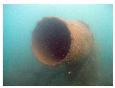
Figure 112: Outfall diffuser for discharge of brine (file photo: HMR Consultants)
