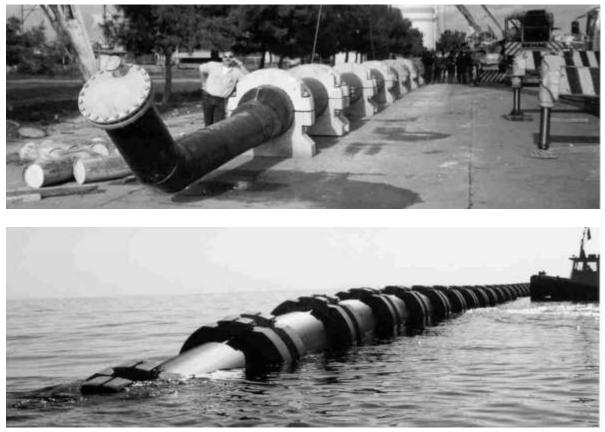
Figure 21: Antalya wastewater outfall (Turkey) during installation in 1997. *Top*: Diffuser section assembling on shore. *Down*: Feeder section ( $L_F = 5$  km, HDPE pipe, D = 1600 mm) while sinking with attached concrete weights on the seabed (PipeLife Company)
