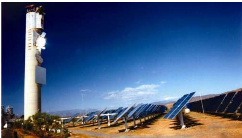
*Fig. 3. The CESA-I facility seen from the East with heliostat rows focusing on the medium-height test level (60 m.)*
