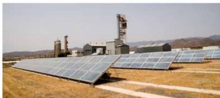
*Fig. 17. PSA SOL-14 MED Plant (left), double-effect LiBr-H<sub>2</sub>O absorption heat pump (upper right) and 500-m<sup>2</sup> CPC solar collector field (bottom right)*
