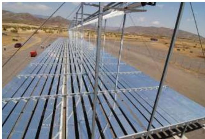
*Fig. 8. Photo of the linear Fresnel concentrator erected at the PSA*
