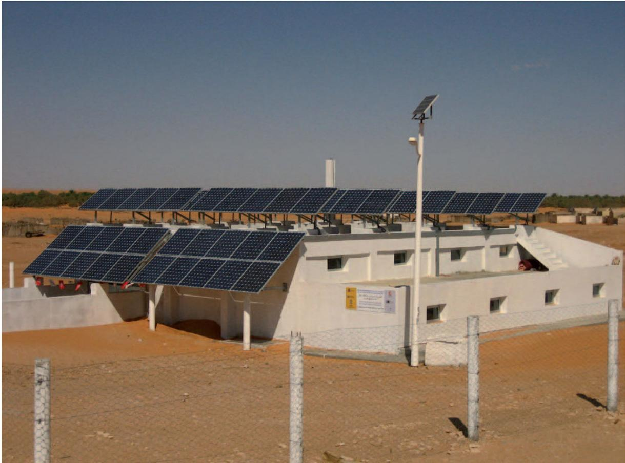
Figure 23: A 2.1 m<sup>3</sup>/h nominal capacity brackish water PV-RO plant in Tunisia, installed by the Canary Island Institute of Technology, Spain.
