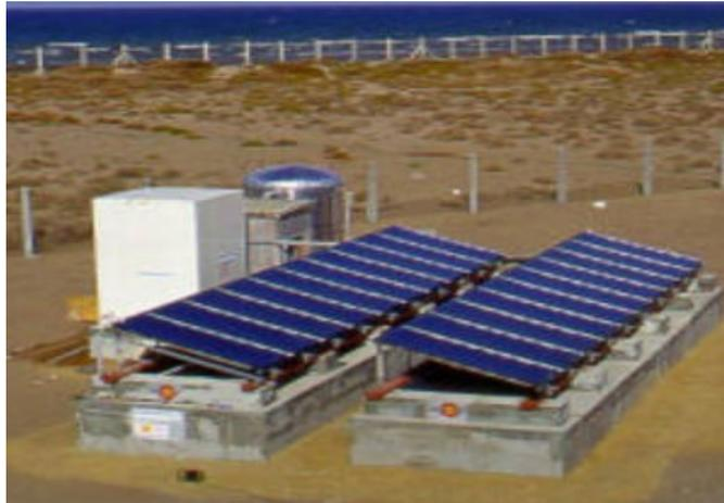
Figure 20: A 1 m<sup>3</sup>/d multiple effect HDH unit in Oman
