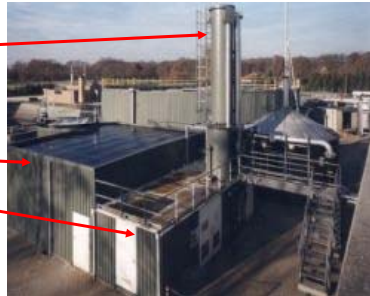
THIOPAQ®- Bioscrubber for H 2 S removal from biogas produced in papermill UASB, The Netherlands
