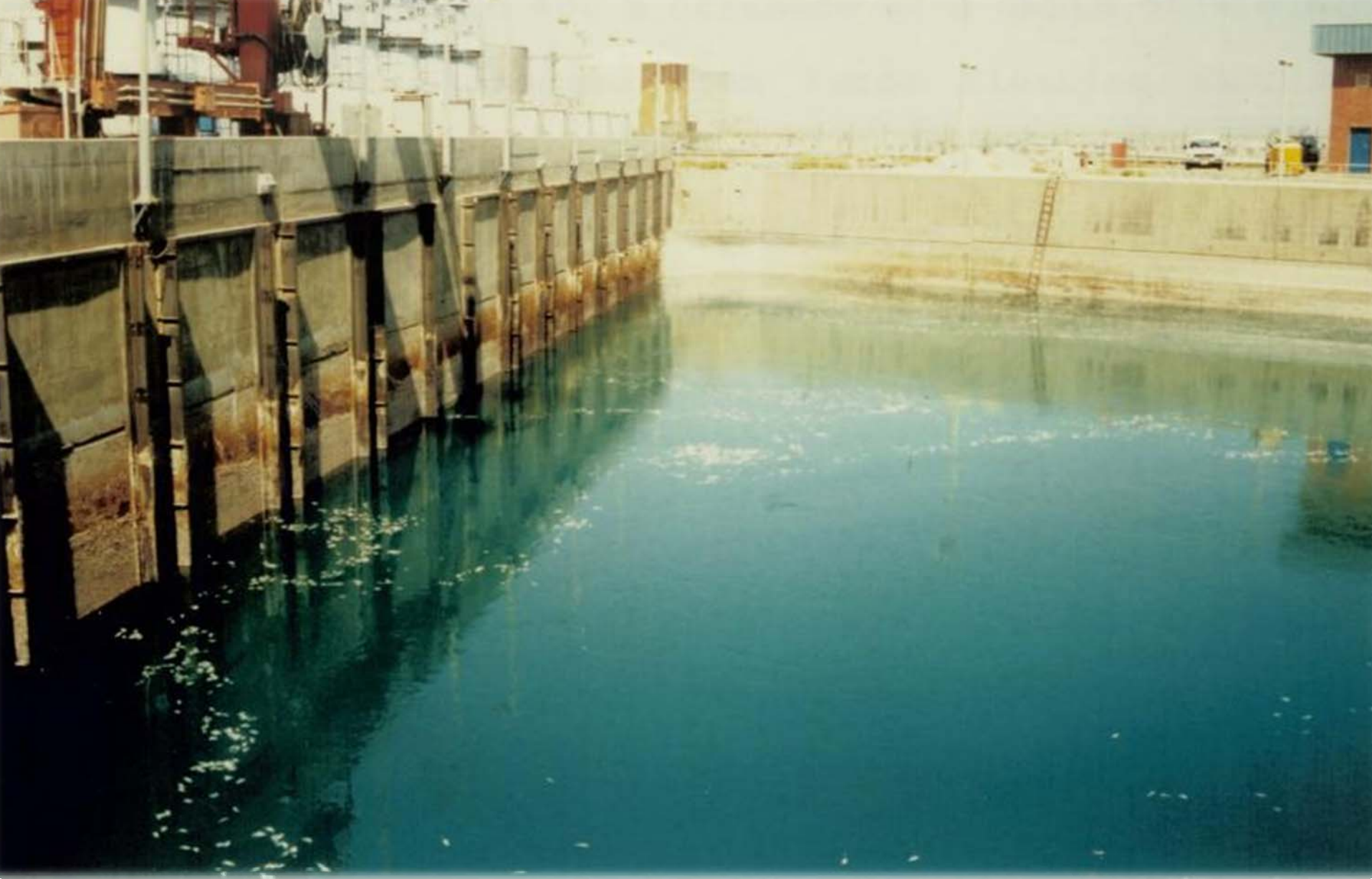
Forebay of a desalination plant intake
