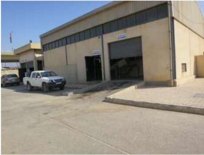
Figure 18 Screen house odour control futile with large open doors
