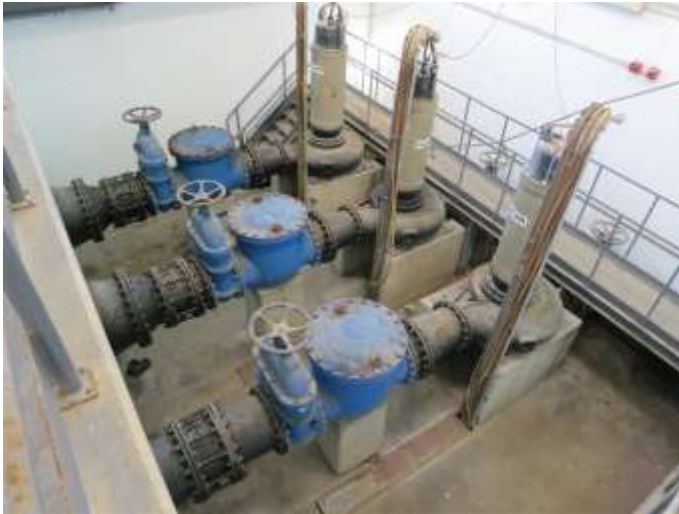
Figure 10 Outfall pumps
