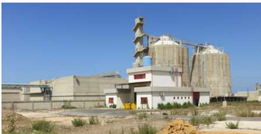
Figure 20 Anaerobic Digesters on Solid waste treatment facility next to WWTP
