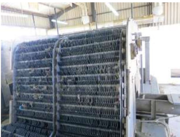
Figure 4 Tooth raked fine screen
