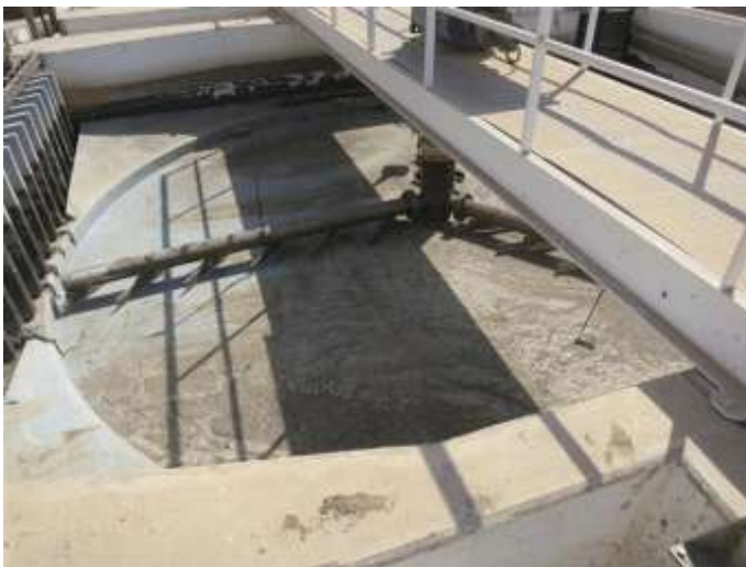
Figure 7 Drained Grit Detritus tank
